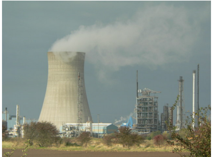
Cooling towers are often associated with nuclear plants, but this familiar design is also used at natural gas and other thermoelectric power stations. This tower serves the Saltend Power Station in East Yorkshire, a combined-cycle natural gas plant that supplies electricity and steam for nearby industries.
