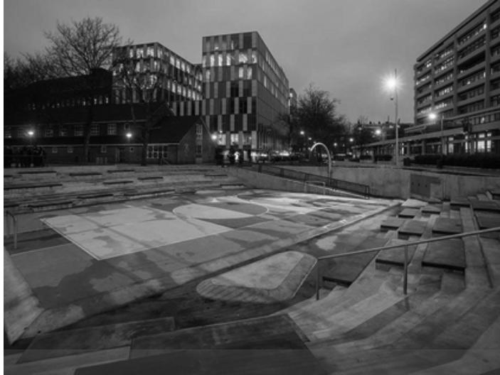
Flash floods are a challenge for urban areas with impervious concrete surfaces. Bentheplein, a city near Rotterdam in the Netherlands developed a solution called "Waterplein" (water square). When heavy rains occur, stainless steel gutters channel water into one of three retention ponds, the largest of which only fills with extremely heavy rains. When dry, which is most of the year, the ponds can be used as amphitheaters, basketball and volleyball courts, and skateboarding.
