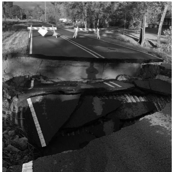
Flash floods very often cause extensive and expensive damage to infrastructure such as roads and bridges. This is damage from a flash flood to a roadway located in Fort Payne, Alabama in 2022. Storms brought 15-20 inches (38-51 cm) to southeast Alabama, causing widespread destruction.
