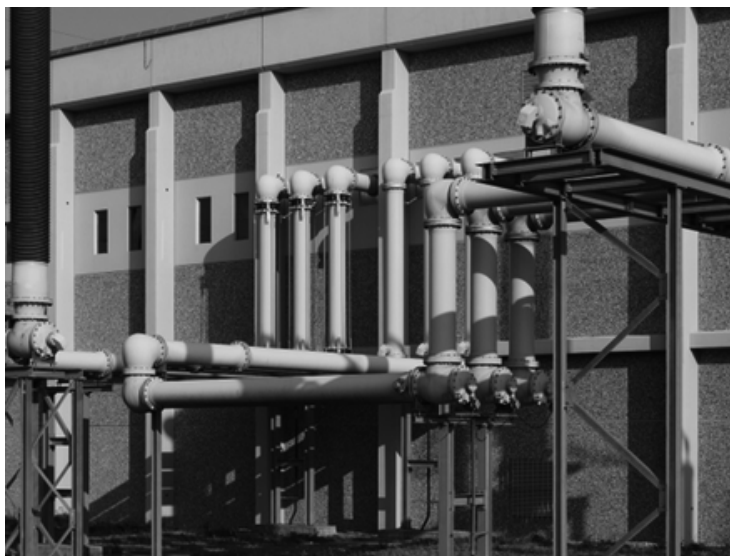
High-voltage power lines at the Leingarten substation in Germany use sulfur hexafluoride (SF 6 ) gas as an insulator. SF 6 is commonly used in electrical systems for its ability to prevent short circuits and safely handle high voltages.
