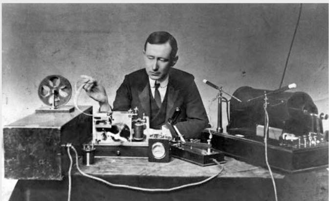
Engineer and inventor Guglielmo Marconi demonstrates his spark-gap transmitter, used in his first long distance radio transmissions during the 1890s.
