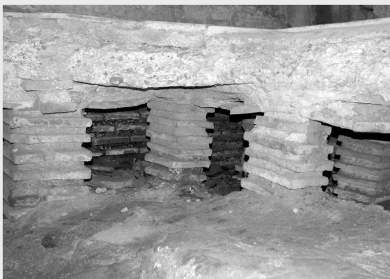
Ancient Roman floor heating (hypocaust) in Ostia Antica, southwest of Rome.
