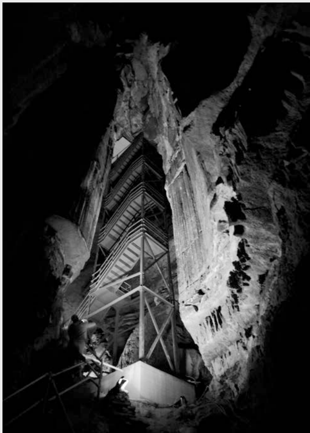
Staircase tower in Mammoth Dome, Mammoth Cave, Kentucky. This vertical shaft is the connector between the lower-Historic trail and the upper-Historic trail. In 2008, this 190 ft (58 m) tower replaced a 53-year-old structure. The new tower allows visitors to make the 2-mi-long, 2-hr-long Historic tour a loop route with minimal retracing of their path.
