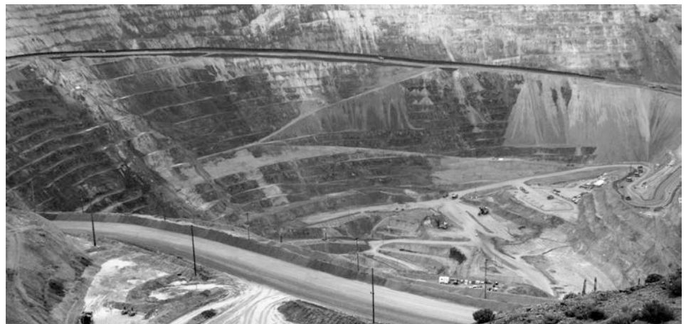
The Bingham Canyon copper mine in Utah has produced more than 12 million tons of porphyry copper. The mine is more than 4 km (2.5 mi) across at the top and 800 m (0.5 mi) deep—large enough to be visible from space. It is one of the engineering wonders of the world.
