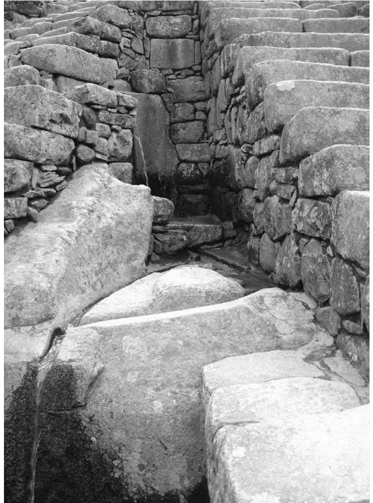
Water distribution and drainage systems took advantage of the natural plumbing of faults and fractures in the city.
