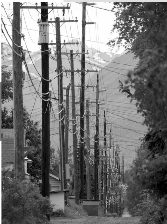
Power transmission lines near Anchorage, Alaska.
